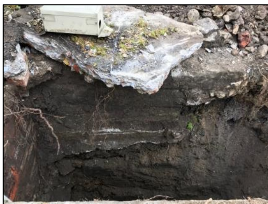
Plate 1 Concrete wall supports
